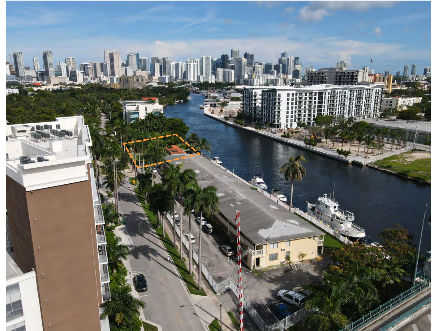
Aerial photo of site looking east
